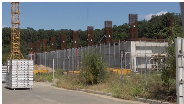
(b) Photograph of the building (2026.08.28)
