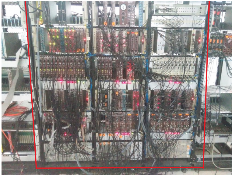
The old RoSphere acquisition system. It's size and impressive number of modules are readily observable. It only recorded signals from 50 channels – Source: Photo taken by the author
